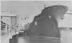
"Esso Malacca" on June 28 took the first cargo of 135,000 barrels of C450 low sulfur fuel oil processed by the new HDS units to West Palm Beach for discharging into Humble's tankage.
